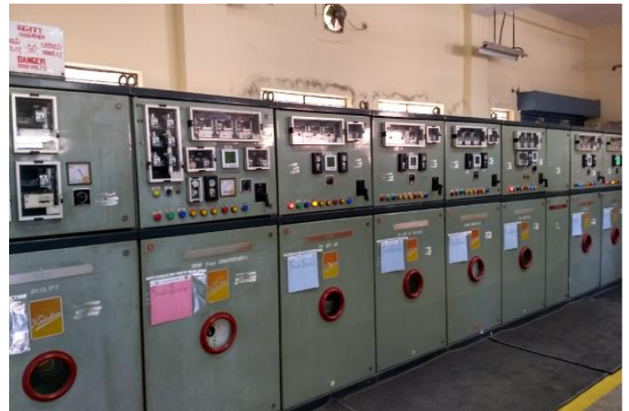
Figure.6. Typical smart meter installation (at 66/11kV SS)
