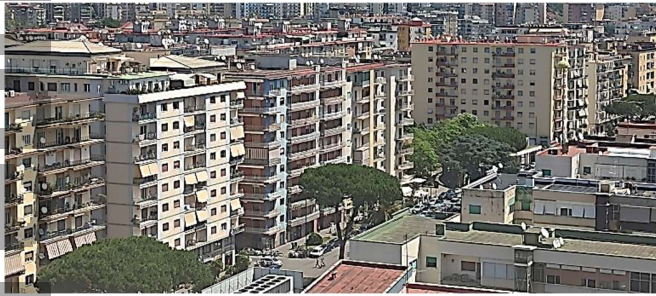
Fig 1 The building typology (multistory, reinforced concrete frames and hollow blocks for walls and ceilings)
