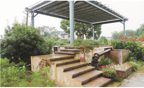
Fig 1 Distributed solar PV plus tourism (A PV station hidden in the beautiful wall painting)
