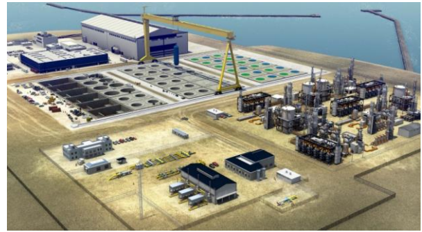
Figure 4. Hydrogen Gigafactory with Factory in Back, Reactor Field in the Middle and Hydrogen Plant in the Front (Courtesy of LucidCatalyst)
