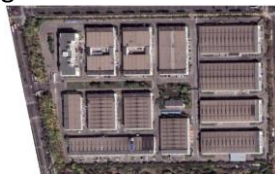
Fig.3 The intelligent unmanned equipment industrial park
