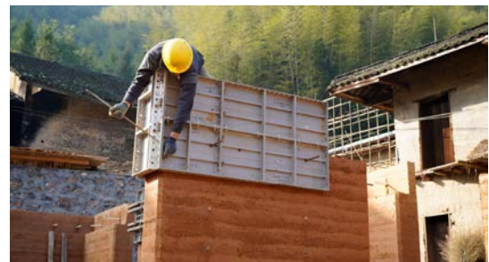
Fig. 11 photo by CCMCCF, rural rammed earth house construction in China
