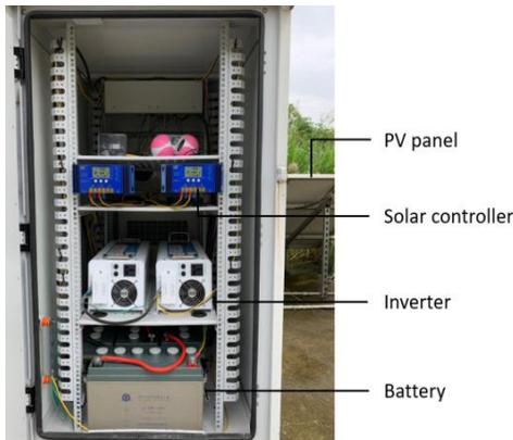
Fig 2 PV power generation system.
