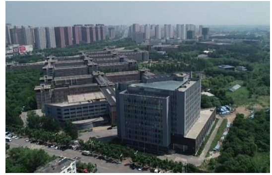
Fig. 1 Real photo of engineering training center
