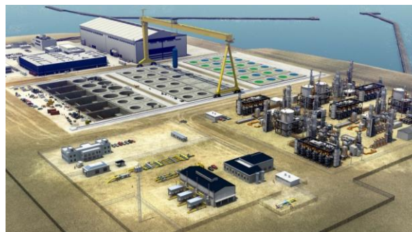
Figure 4. Hydrogen Gigafactory with Factory in Back, Reactor Field in the Middle and Hydrogen Plant in the Front (Courtesy of LucidCatalyst)
